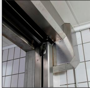
A central point of the standard is the ease of cleaning the surfaces and construction elements. Attention was paid to slanting surfaces on which no water or waste can collect.
